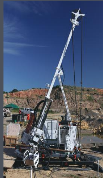
Surface Coring Rigs
